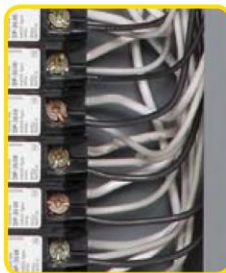
▲ Pigtail Neutral connection
