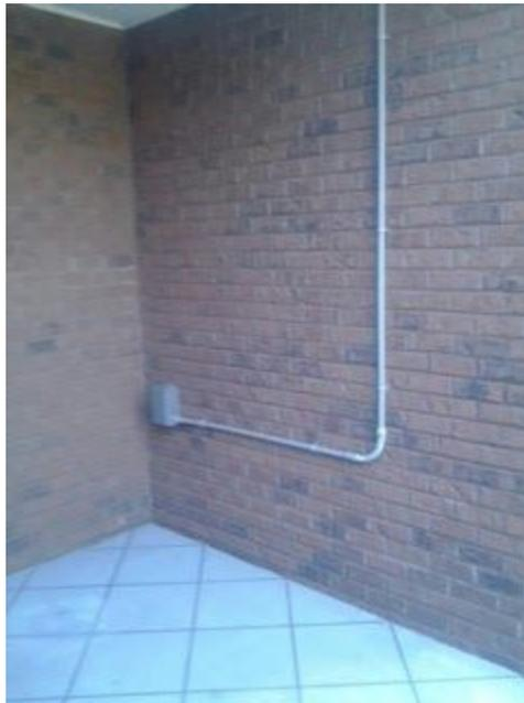
This is an incomplete installation and is not acceptable for the day of delivery. The line to the spa is missing. See below two examples of this line, which is called the whip.
