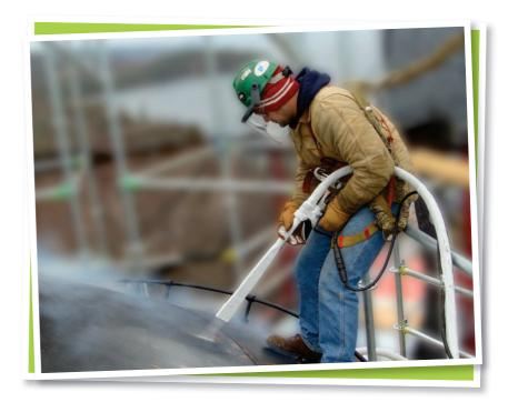
CDG specifically liked the fact that dry ice blasting promoted itself as a method that can clean electric components and will not harm them. Another major factor was that dry ice blasting produces zero residue, unlike soda blasting, and does not generate any secondary waste.
