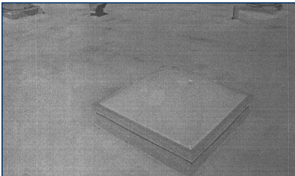
The skylight has been damaged by hail, but the SPF roof exhibits no visible signs of damage.
