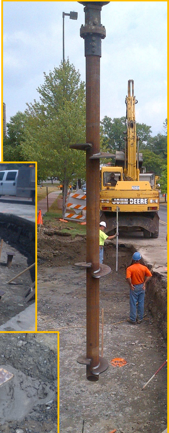
Filling piles with Concrete
