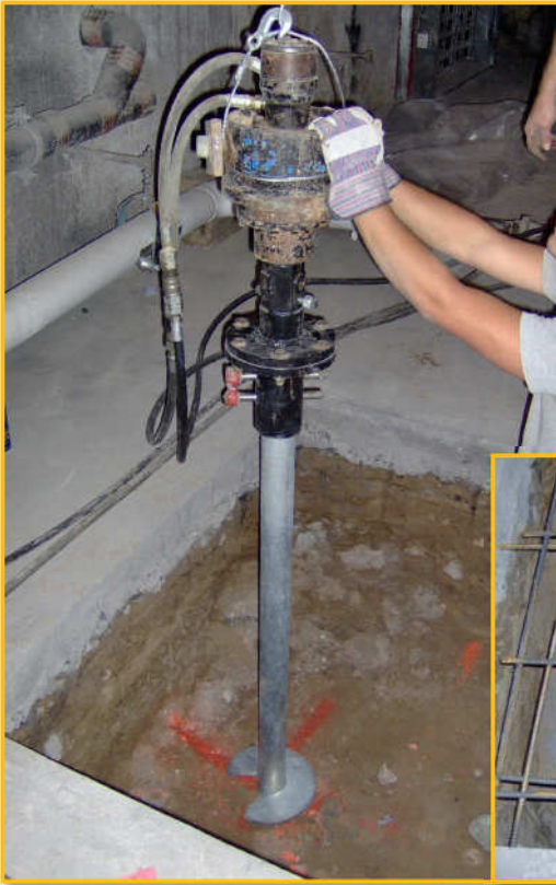
Installing piles in basement of University for new column support...
