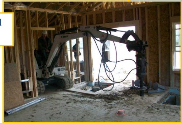
Interior Floor and Wall Support
