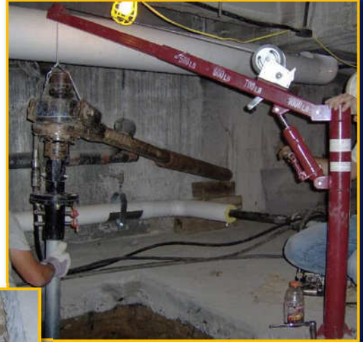
Installing piles in basement of University for new column support...
